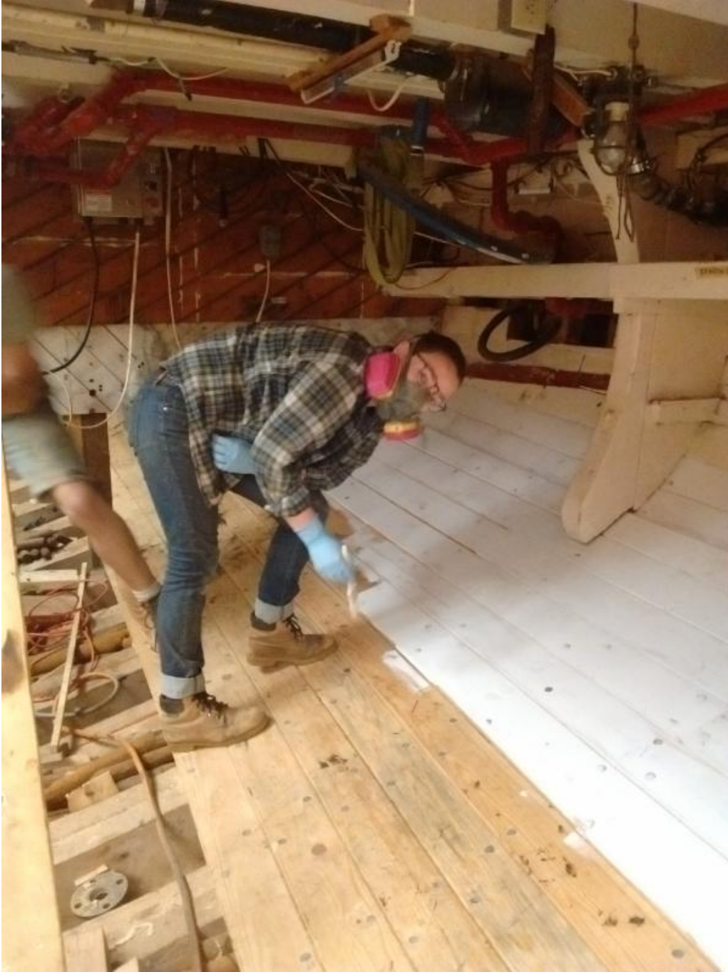
The ceiling is being painted.
