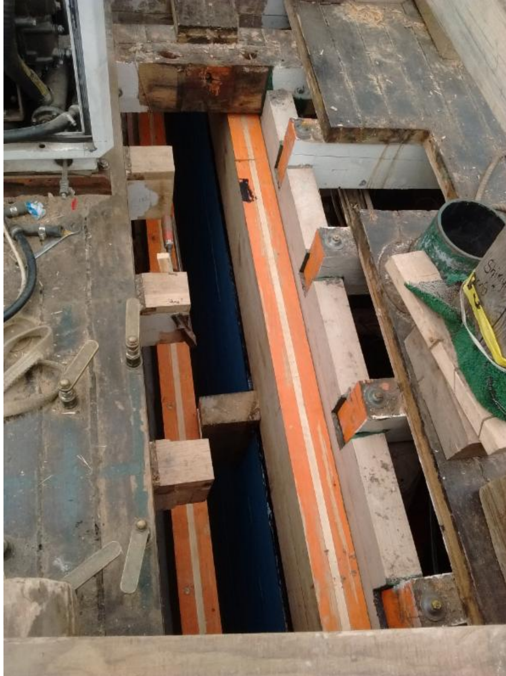
The centerboard trunk has almost reached the deck!
