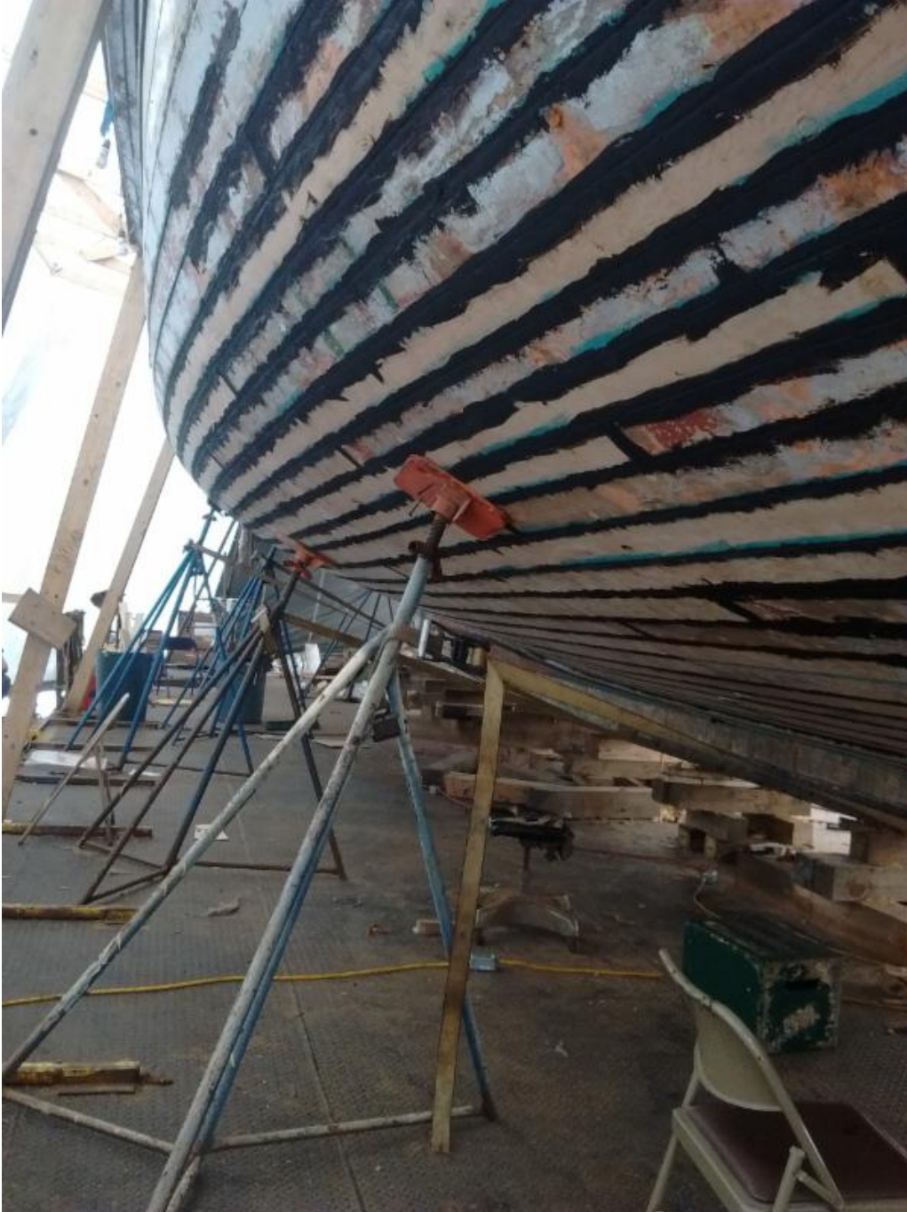
All seams are finished on the starboard side.
