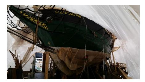
The port bow of the sloop. All the planks and frames below the waterline in this section were replaced in 2010. The above the waterline portions will need to be replaced in the next five years.
