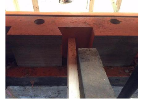
The inboard frames will be tenoned into the mortises in the bedlog where the piece of 2x6 is in the photo.
