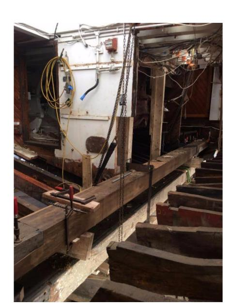
Last week we brought the keelson section up inside the hull. Now that's it's fit the right way, we're making sure we have the tools to fasten it in place. It will have to be removed again in order to install the starboard bedlog beneath it.
