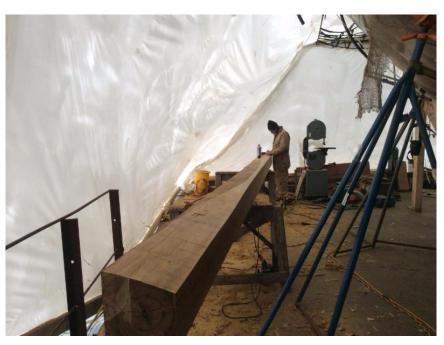
The port lower bedlog is the base of the port side of the centerboard trunk. It also forms part of the hull, so it has a lot of shape to it.
