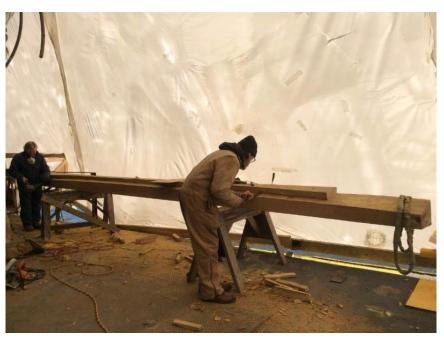
Here, shipwrights cut the rabbet where the hull planking will fasten, creating a watertight joint.
