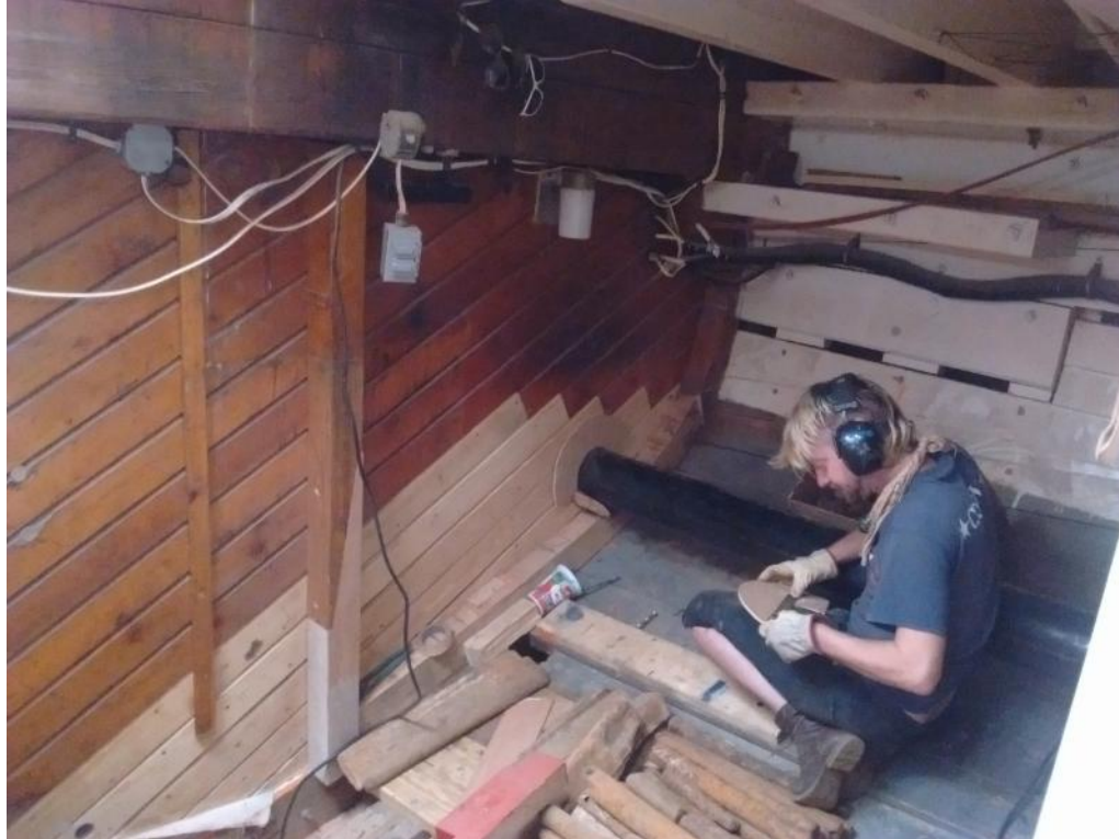
Shane is working on the exhaust supports.
