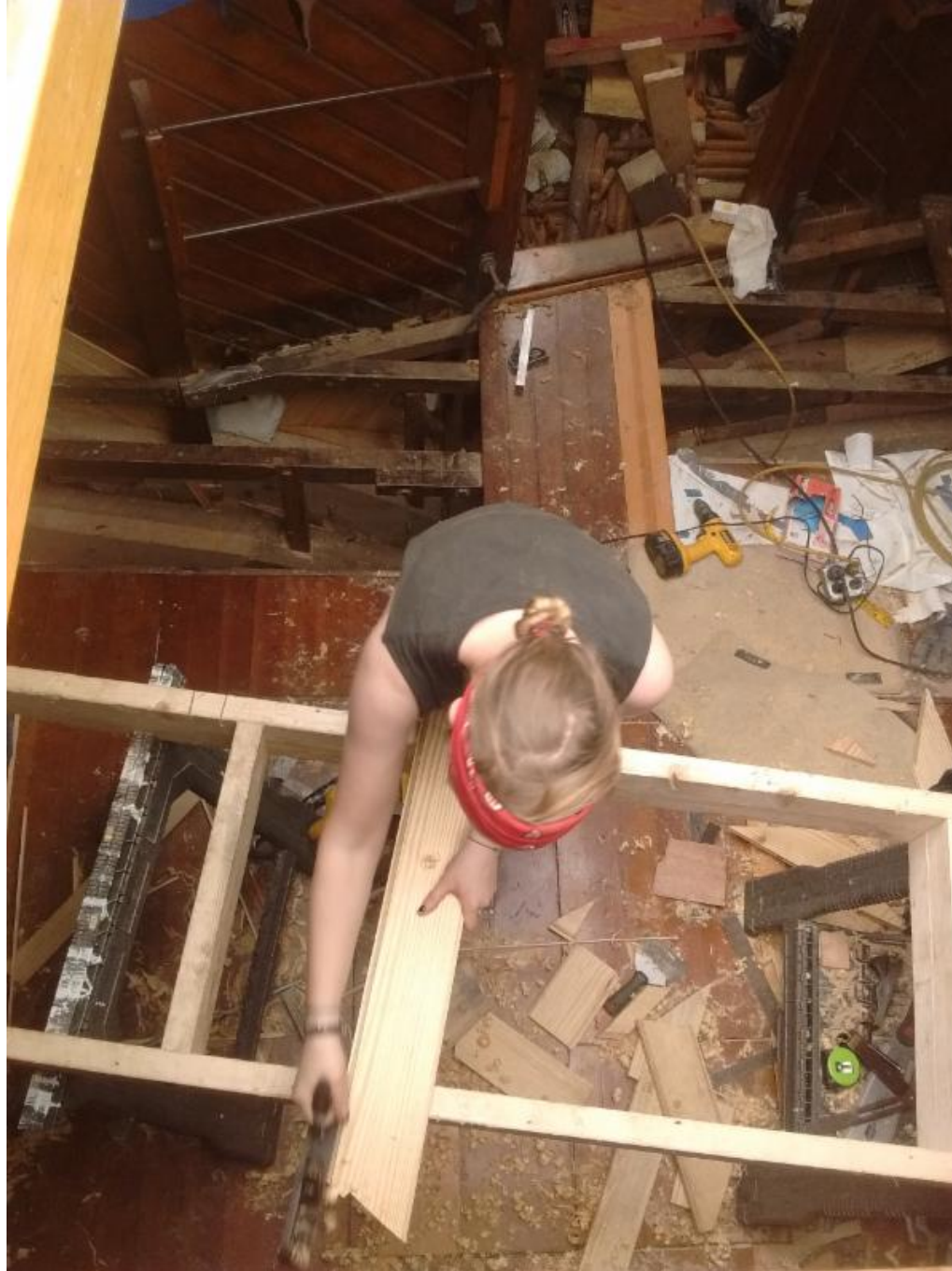
Catherine Rose is working on putting the bulkheads in place.
