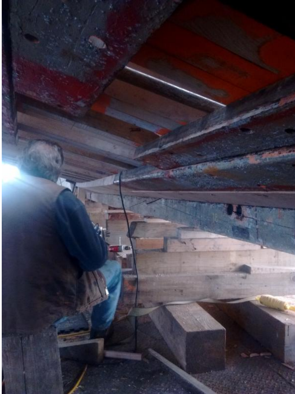
The starboard side garboard and broad strake.
